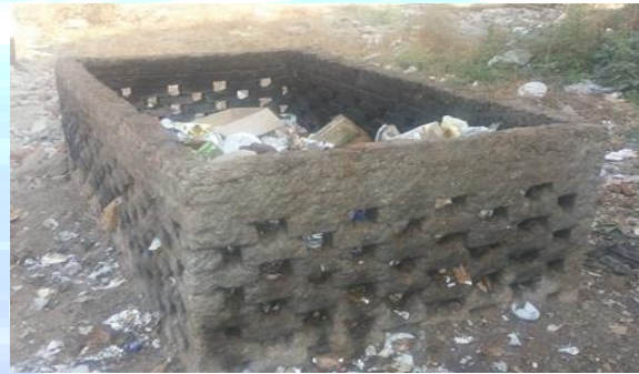
Construction of NADEP method of compost
