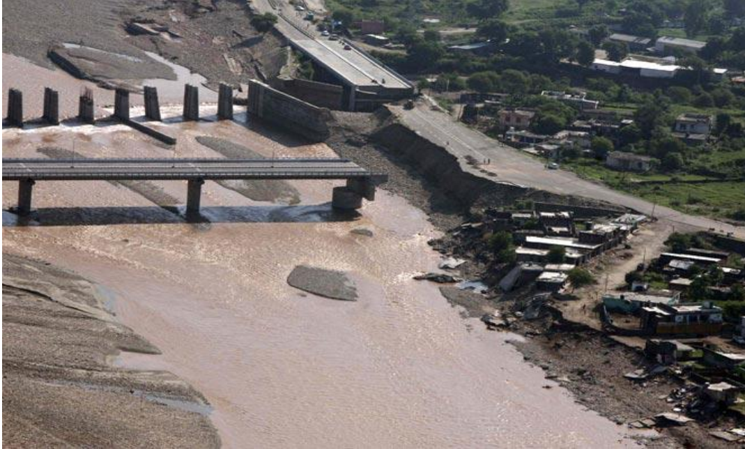
An aerial view taken from an Indian Air Force's helicopter shows the remains of a bridge at Beli Charana after it was swept away by floodwaters from the river Tawi on the outskirts of Jammu.
