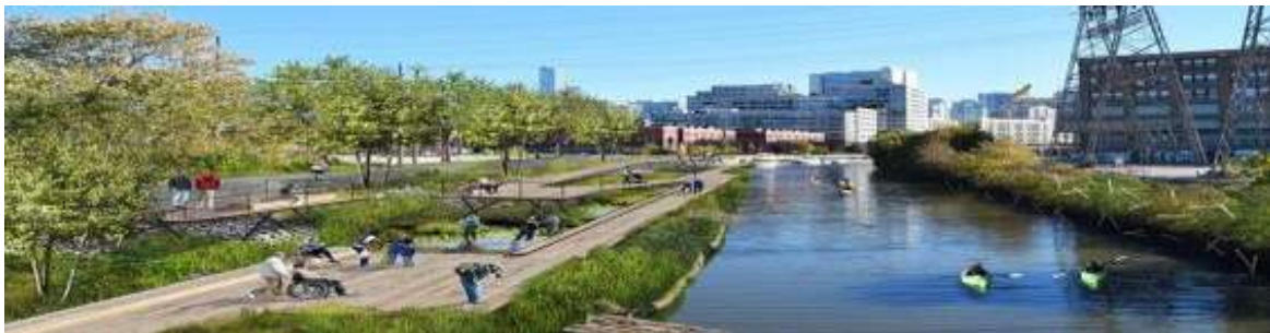
Fig.1 Built components and open spaces at the riverfront forming a balanced urban weave.
