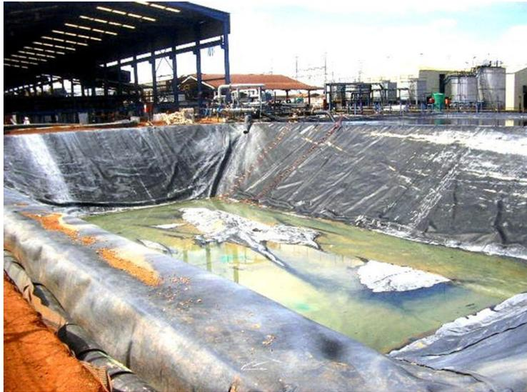
**Figure 11 : Geomembrane depleted electrolyte pool**
