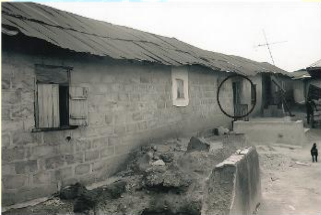
Figure 1: Sandcrete and Coursed Earth Mix; Baale Aguodo Compound (High Residential Density Zone).
