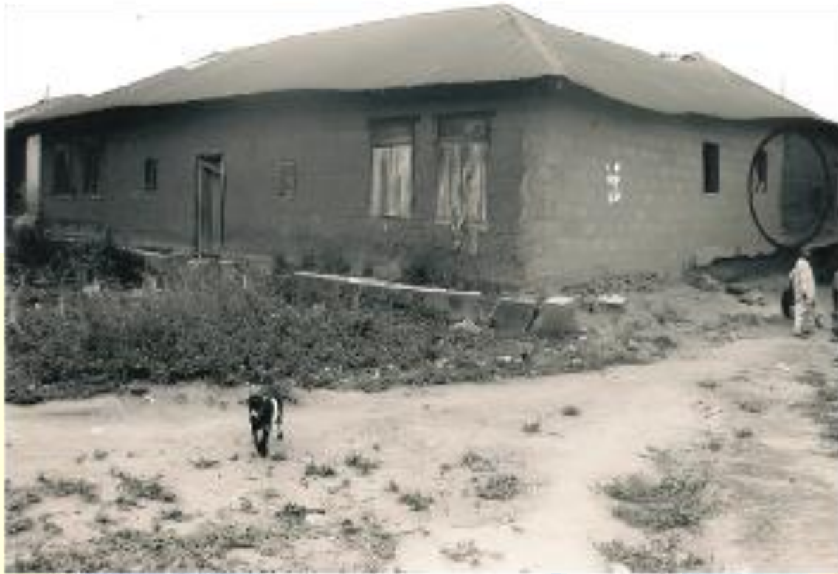
Figure 3: Back of Apaina Compound, Masifa Area, Ogbomoso: (Coursed Earth with Sandcement blocks).
